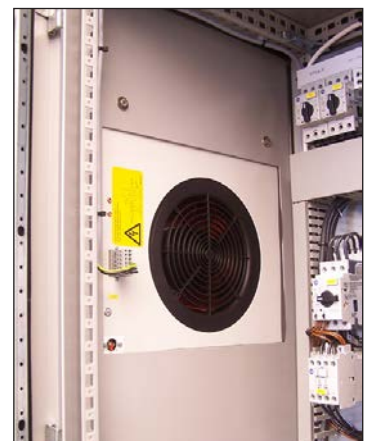
Fan, aspirating warm air out of the electric cabinet
