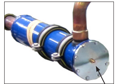
Filter drier, service valve
