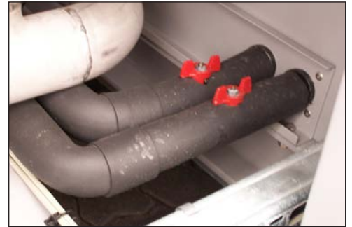
Chilled water lines to the evaporator in the refrigerant section with open stop valves
